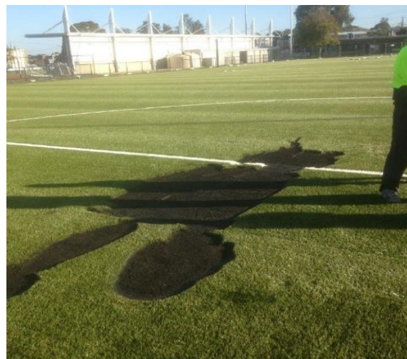
Photo 8: Vandalism can entail a whole section being cut out and replaced
