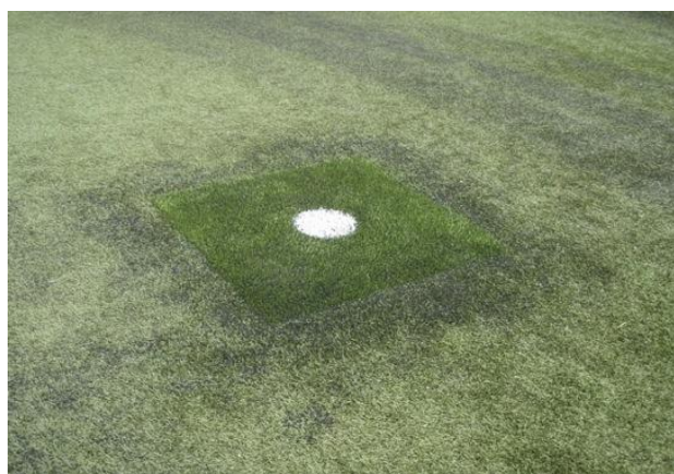
Photo 11: Replacement penalty spot due to excessive wear
